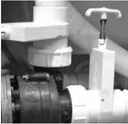
Slice Valve and Pump Union
