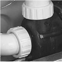
Vent air by slightly opening pump unions.
