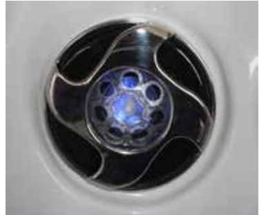
Figure shows Jet installed
