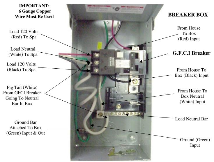
NOTE: The White Neutral Wire from the GFCI MUST be connected to an incoming Line Neutral. The internal mechanism of the GFCI requires this Neutral connection. The GFCI WILL NOT WORK WITHOUT IT.
