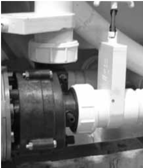
Slice Valve and Pump Union
