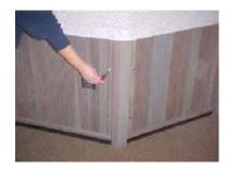
Install corner posts (pay attention to "up" arrows) to side panels, then small panels to each corner post around spa using panel bolts and bolt driver.
