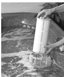
1) Center filter cartridge over canister
